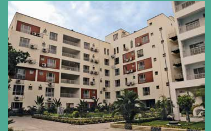
MEGHALAYA HOUSE, RUSSEL STREET
